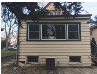
8316 N. KILDARE AVENUE BACK (WEST ELEVATION)
