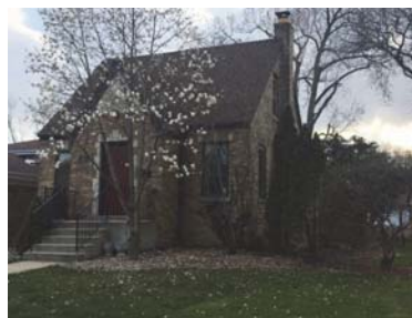
8316 N. KILDARE AVENUE FRONT (EAST ELEVATION)
